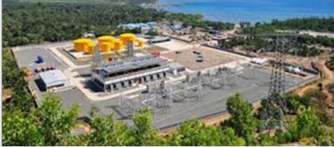
Betano power plant - 136.6 MW (8 units of Wartsila's W18V46 engines);
