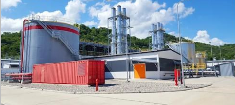
Betano power plant - 136.6 MW (8 units of Wartsila's W18V46 engines);
